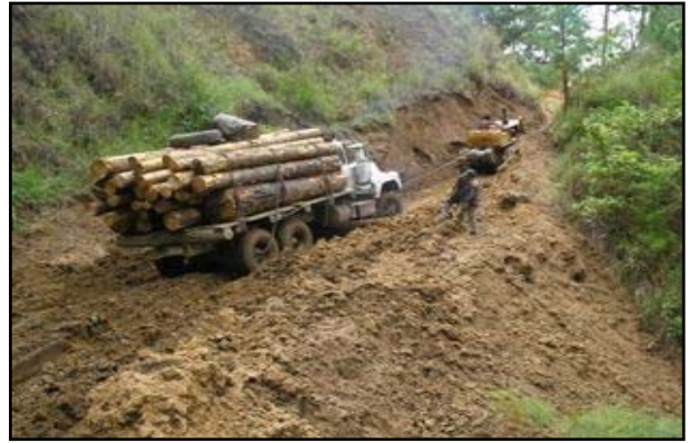
Picture 4: lack of engineering works in road building
